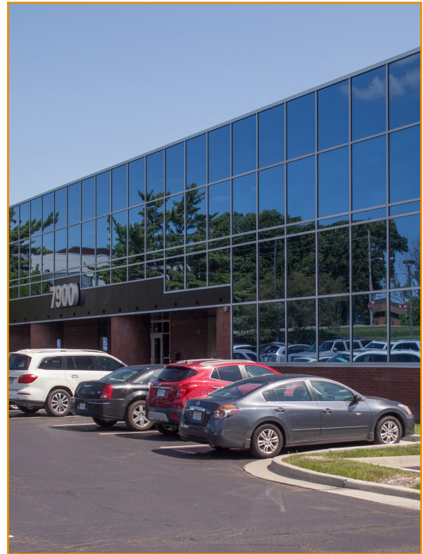
All New Exterior Curtain Wall Glass
